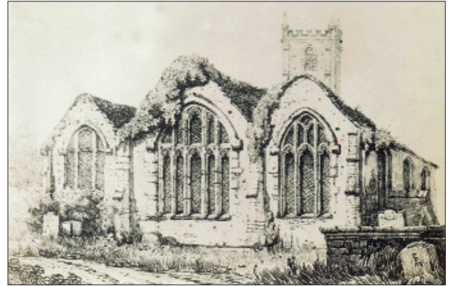
Northlew church before the restoration was overgrown, with the roof covered in ivy; the churchyard was grazed and trampled by sheep and oxen and soil from graves was piled up against the walls
