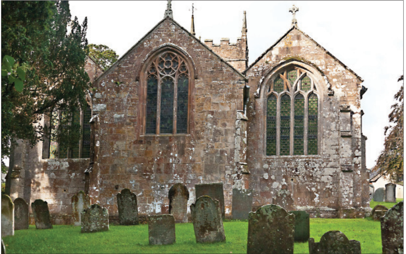
Present day view of the east end of the church - spot the difference
